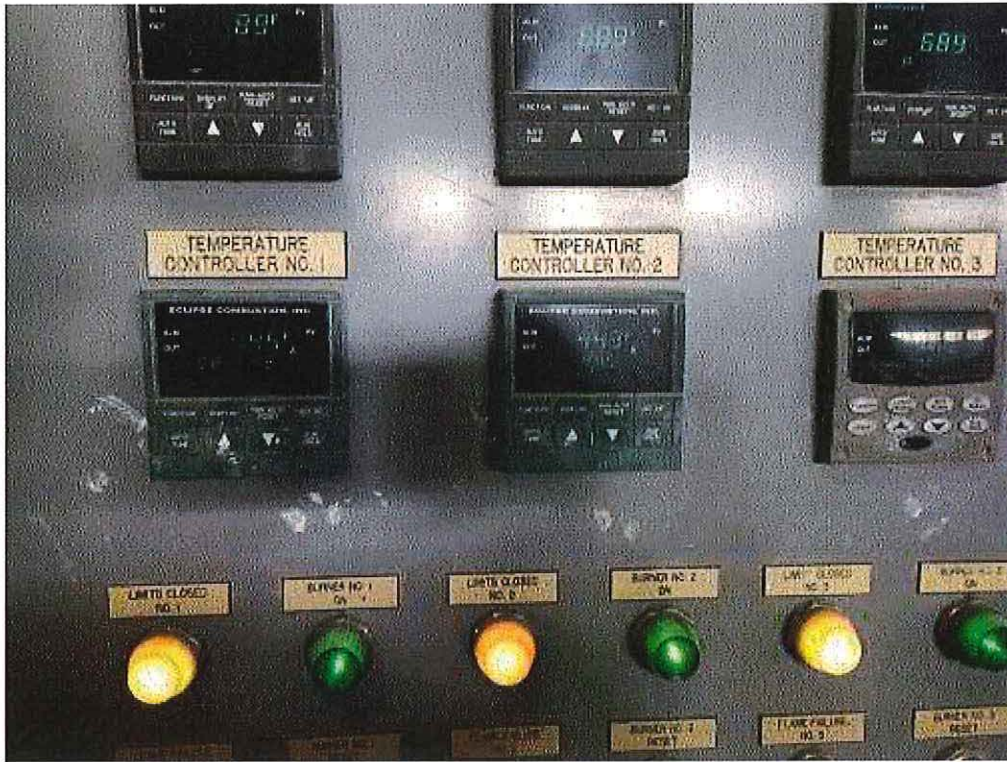
Image 4(BMH Dryer) : Device to monitor and control the temperature of the BMH dryer in EUNEWCUSTOMLINE.
