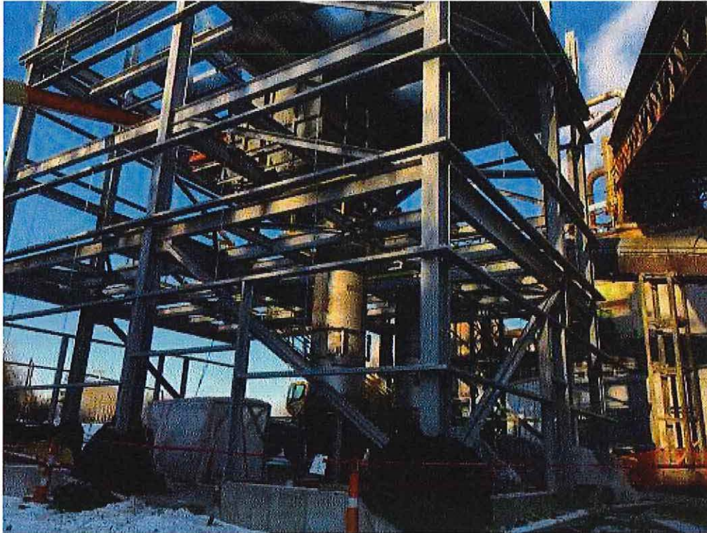
Image 1(FG-PERLITE EXPAND) : Construction of new perlite expander furnaces.
