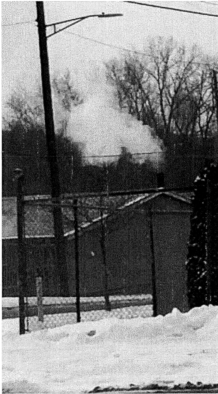
Image 3(smoke 2) : Zoomed in photo of smoke stack. Also taken nearby complainant location; NE of Michigan Ladder.
