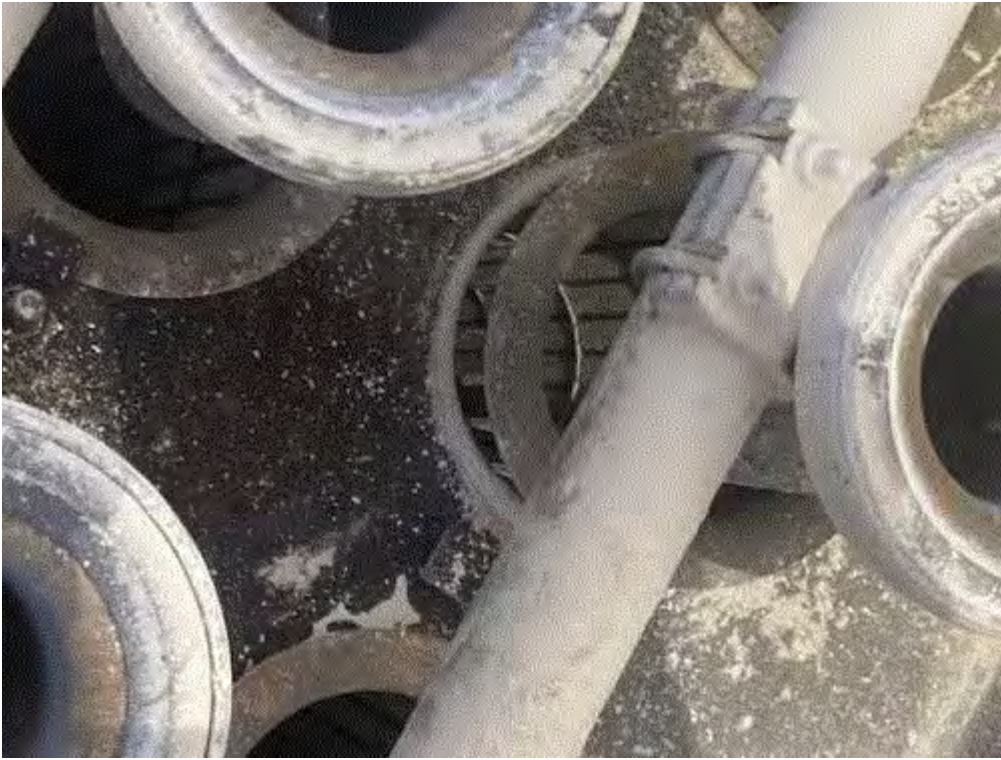
Image 8(Unsealed bags) : Photo credit: Michigan Brick. Photo before sealer was applied to bag seals.
