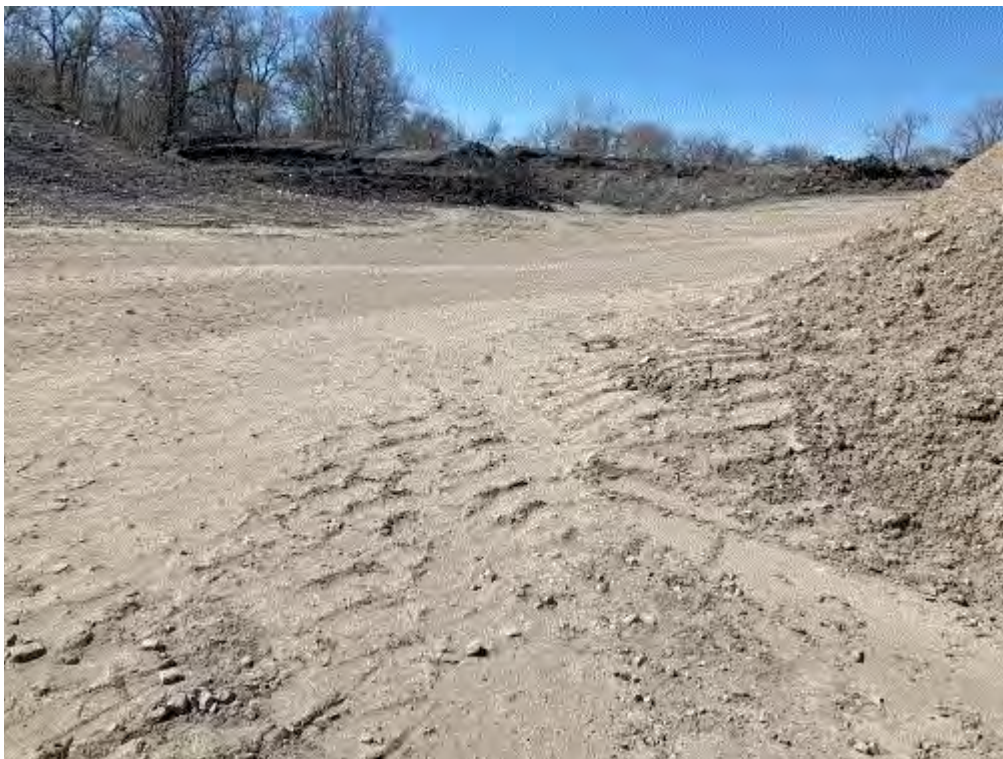
Image 5(Dry haul road) : Dry haul road resulted in fugitive dust from truck traffic during inspection.
