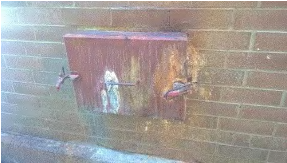
Image 4(Cooling Tower Door) : Cooling tower door (where ambient air is let into cooling tower to maintain a safe temperature for the baghouse). Closed during inspection. Photo Credit: Bill Stevens, Meridian Brick
