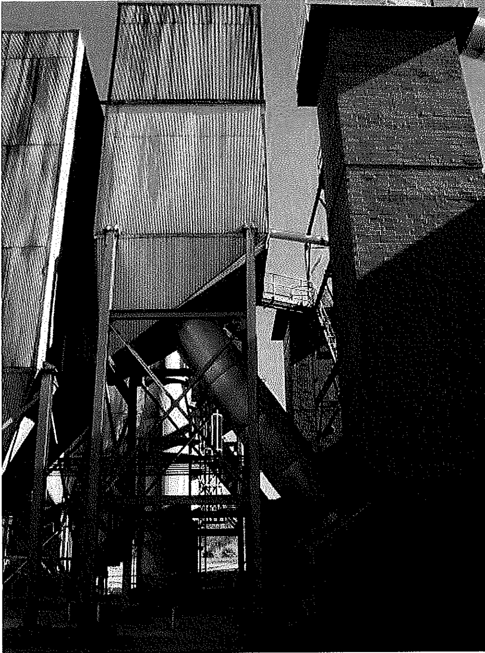
Image 2(Cooling Tunnel) : (Center structure). Lime-laden exhaust air sent to cooling tunnel to be cooled prior to entering baghouse.
