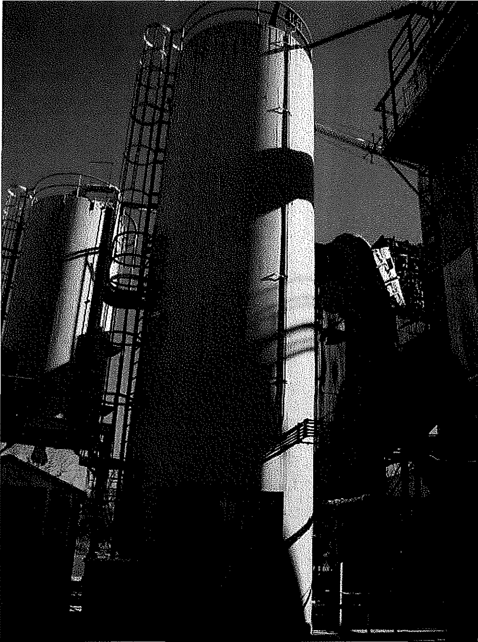
Image 4(Lime Feed Tower) : Lime is stored and transferred from this location into exhaust stream via piping.
