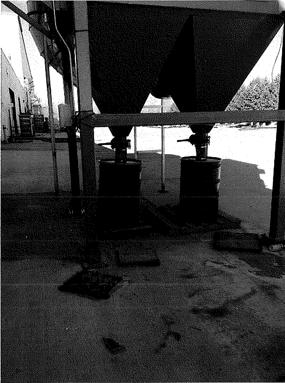
Image 2(Sand Blast Baghouses) : Note the waste particulate from sand blasting on the ground: both the sand blast media itself and the particulate removed from metal parts
