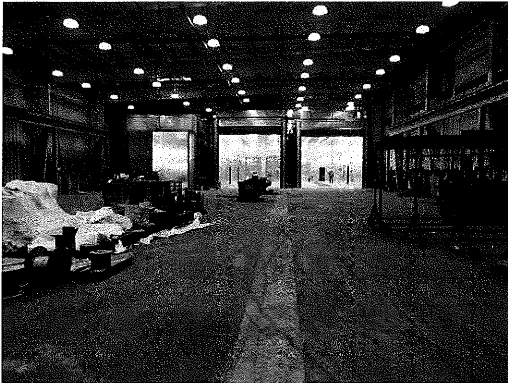
Image 1(New Booths) : L to R: new sand blasting booth, 2 new paint booths for train car coating operations
